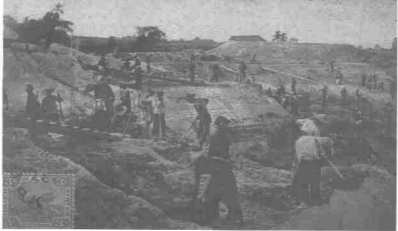
Tin-mining; removing surface soil (Cheras, Selangor).
